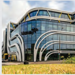
THE MERCURY BUILDING, 33 BROADWAY, NEWMARKET, AUCKLAND
