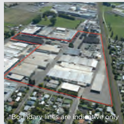
ENZA INDUSTRIAL COMPLEX, WILLIAMS STREET, HASTINGS
