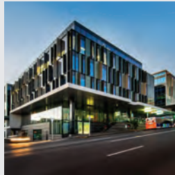
SPARK CITY, BUILDING C, 167-191 VICTORIA STREET WEST, AUCKLAND
