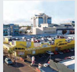
JB HI-FI AND WILSON PARKING BUILDING, 308 BARTON STREET, HAMILTON
