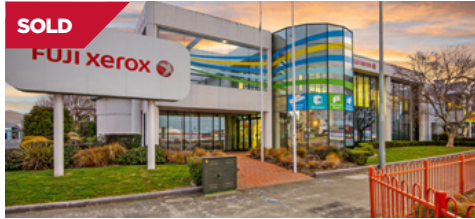
494 Moorhouse Avenue, Waltham
