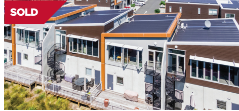
E4/18 Oteha Valley Road Extension, Albany
