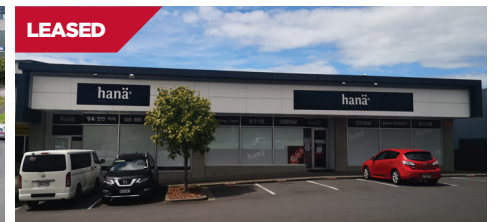
10 and 11/329 Albany Highway, Albany
