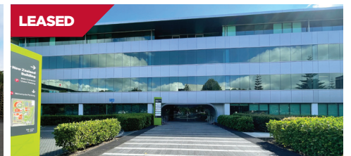
Ground floor, 68-76 Taharoto Road, Takapuna
