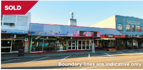
94-100 Broadway Avenue, Palmerston North
