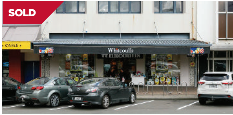
32-36 Broadway Avenue, Palmerston North
