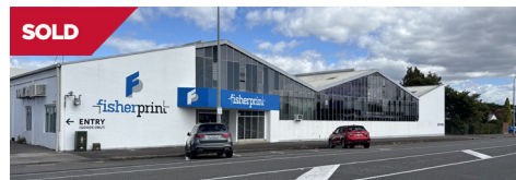
42-48 Cuba Street, Palmerston North
