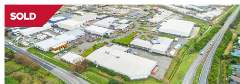
Castle Rock Industrial Park, Christchurch
