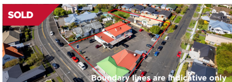
13-15 Great North Road, Whanganui
