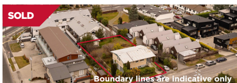
4-6 Hallenstein Street, Queenstown
