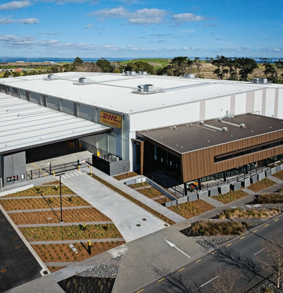
DHL Health Logistics' purpose-built facility on Te Kapua Drive, in Auckland Airport's The Landing Business Park. RDT Pacific managed the entire development process from planning and procurement through to construction and commissioning.
