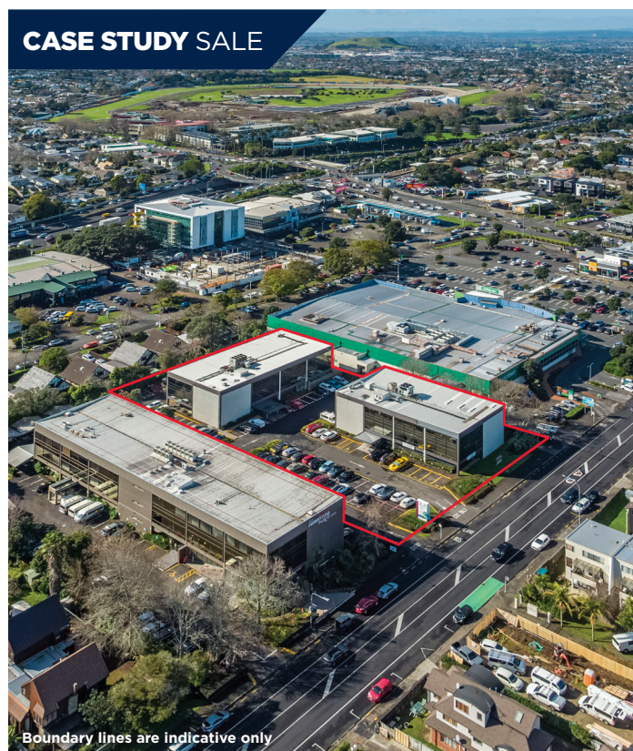
Greenlane 302-308 Great South Road
